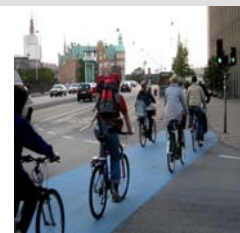
Coloured cross-intersection bike lanes: Do not give cyclists priority, but simply make bicycles more visible to turning vehicles.
