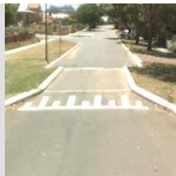
F) Speed bump with road narrowing
